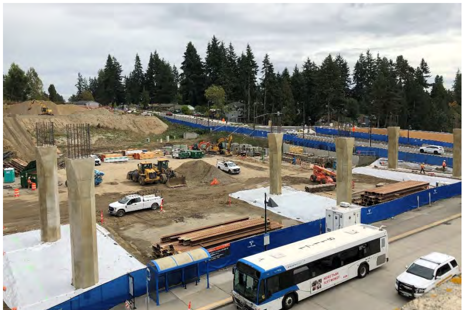
Future Mountlake Terrace Link light rail station under construction
